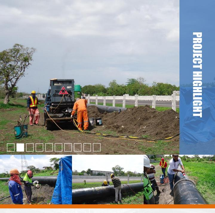
Blasting and Wrapping on Pipe Weld Joint for PGN Pipeline Waru-Manyar
